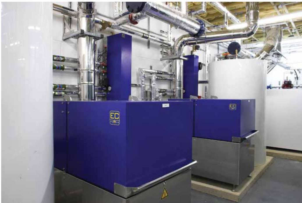
Figure 1: Installation of two LoadTracker CHP systems.
