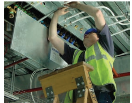
Simple multi-layer pipe installation
