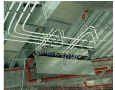
Joint-less continuous AluFlex pipe runs from FloCon module to terminal units
